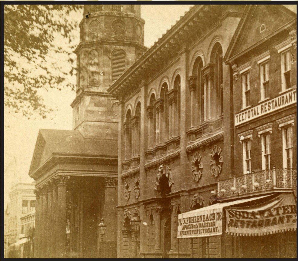
This circa 1860 photograph shows Charleston's Secession Hall and the Circular Church. Both buildings were destroyed in a December 1861 fire. Bob Zeller Collection
